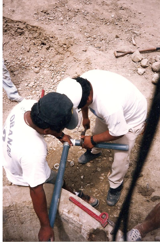
Pictures of villagers excavating the well, installing the surface casing, purging the well, and installing piping for pumping water.
